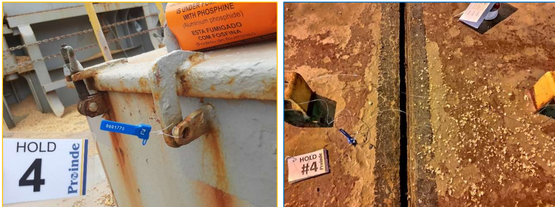
Pictures 53 & 54: Manhole and hatch covers closed on completion of loading of soya beans. Source: Proinde
