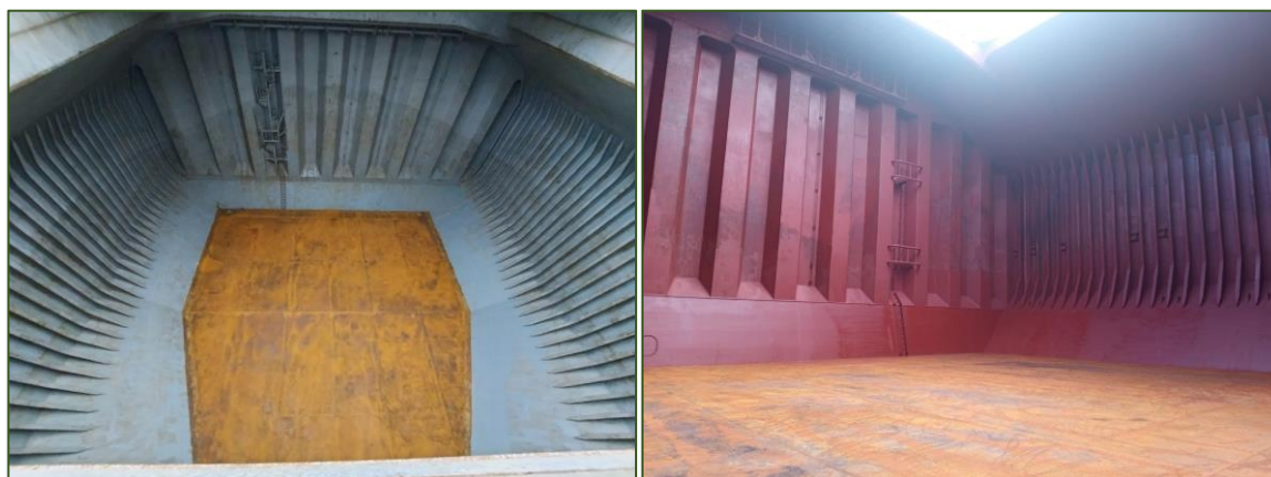
Pictures 19 & 20: Cargo holds during visual inspection. Source: Proinde
